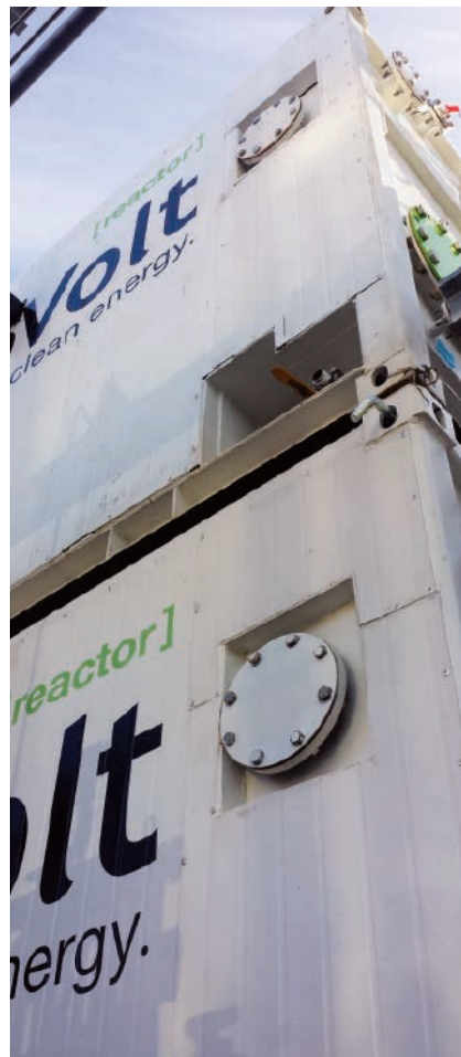
Cambrian Innovation's EcoVolt Reactor harnesses bacteria that produce electrical current and biogas as byproducts of digesting organic matter contained in winery wastewater.
