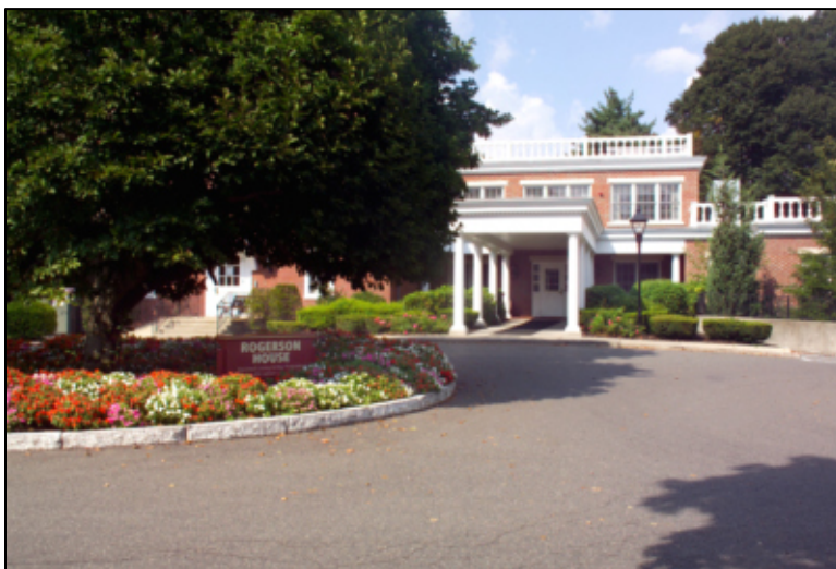
Figure 4. Rogerson House Assisted Living Facility in Boston, MA (Photo: Rogerson House)
